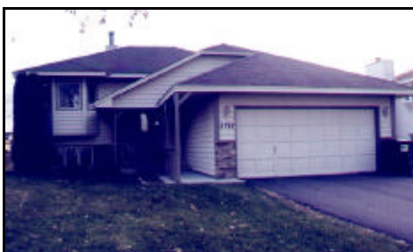
Our Apple Valley House provided by Cedar Valley Church. Thank you CVC!
